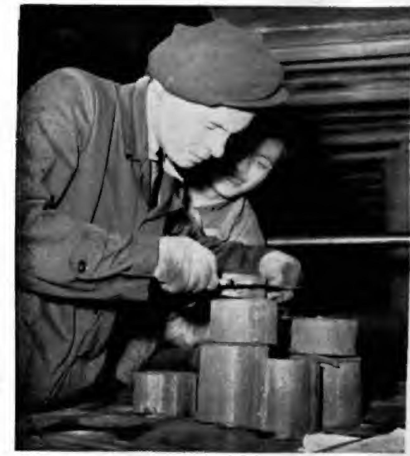
A Soviet expert inspects samples from one of the first batches of structural steel produced by the new mill.
